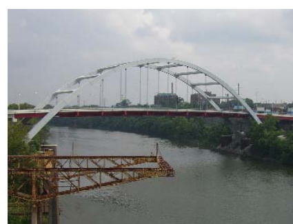
Gateway Bridge; Nashville, TN
