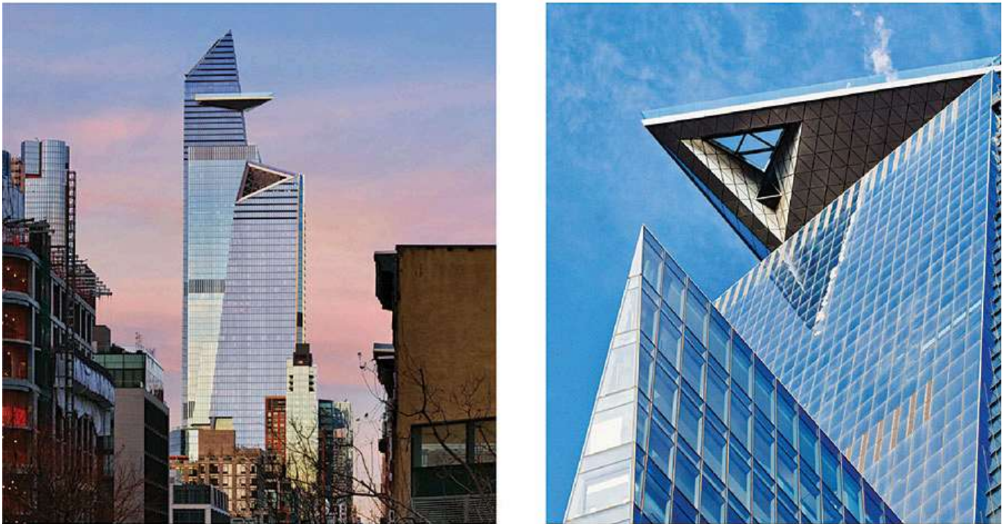
FIGURE 18 Hudson Yards, New York, NY – curtain wall.
