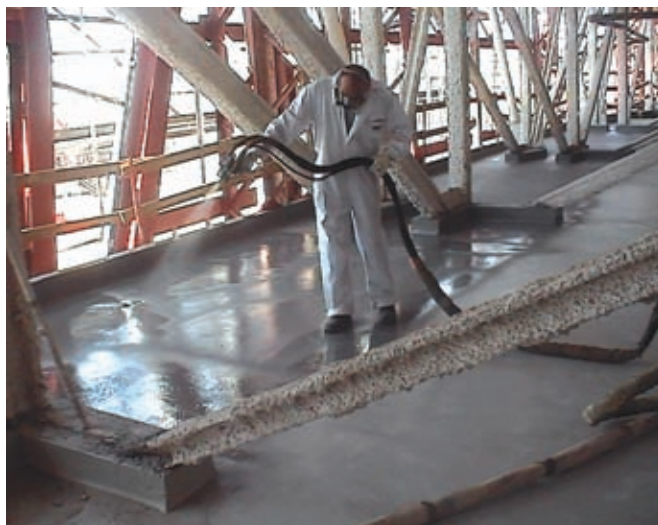
Applying polyurea: Courtesy of DeNeef Technologies (JPCL, February 2005, p. 18)
