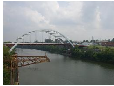
Figure 11-Gateway Bridge, Nashville, TN
