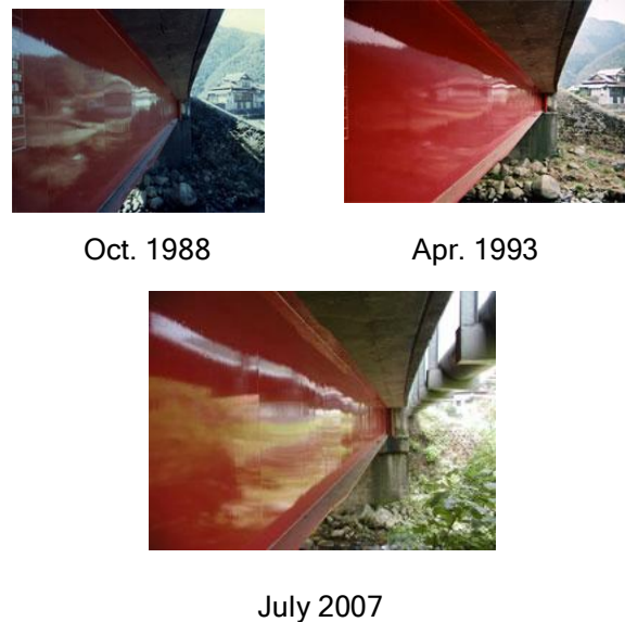
Figure 9-Tokiwa Bridge Over 21 Years
