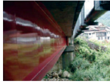
Tokiwa Bridge in 2006, coated in 1987.
