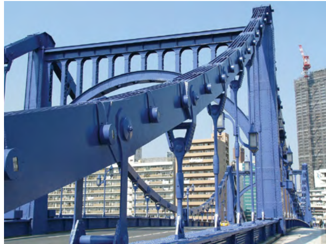
name: kiyosu bridge, japan substrate: steel market: industrial maintenance
