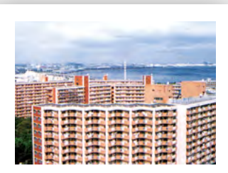
name: mihama estate, japan substrate: fiber reinforced concrete
