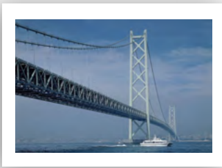
name: akashi straits bridge, japan substrate: steel
