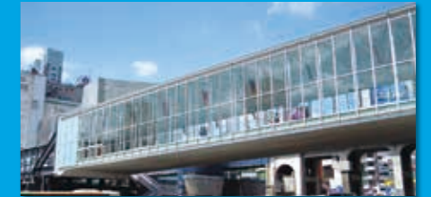
Shibuya Connecting Bridge (Tokyo / 2011)
