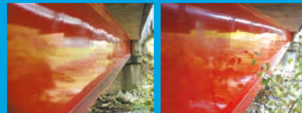
1986 → 30 years → 2016 (Tokiwa bridge in Japan, using solvent type of LUMIFLON™)
