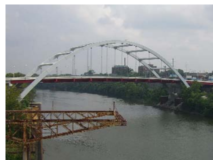
Gateway Bridge; Nashville, TN
