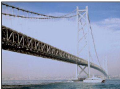
The Akashi Straits Bridge in Japan Courtesy of Winn Dardan
