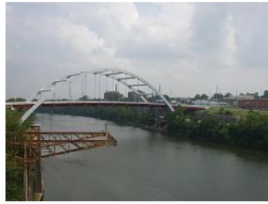
Figure 11-Gateway Bridge, Nashville, TN
