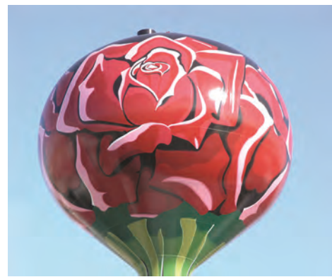
Fig. 2 Fluoroethylene vinyl ether-based topcoat used on the Rosemont Water Tower near the Chicago O'Hare International Airport. Courtesy of Tnemec Company, Inc.
