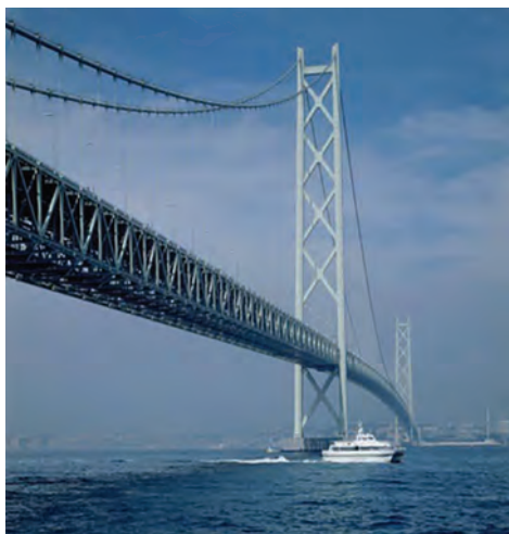
Fig. 1 Fluoroethylene vinyl ether polyurethane-based topcoat used on the Akashi Strait Bridge in Japan. Photo property of Asahi Glass Co. Ltd.
