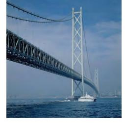
Fig. 1 Fluoroethylene vinyl ether polyurethane-based topcoat used on the Akashi Strait Bridge in Japan. Photo property of Asahi Glass Co. Ltd.
