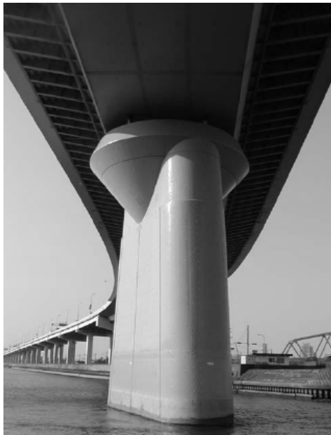
Steel Panels Encasing Concrete, Painted In 2007
