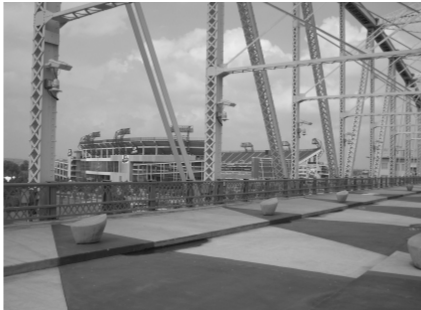
Figure 7. Shelby Street Bridge, Nashville, TN, Photographed in 2006
